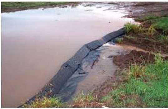
Figure S9. Triangular silt dike (Bulnes Garcia 2013)
