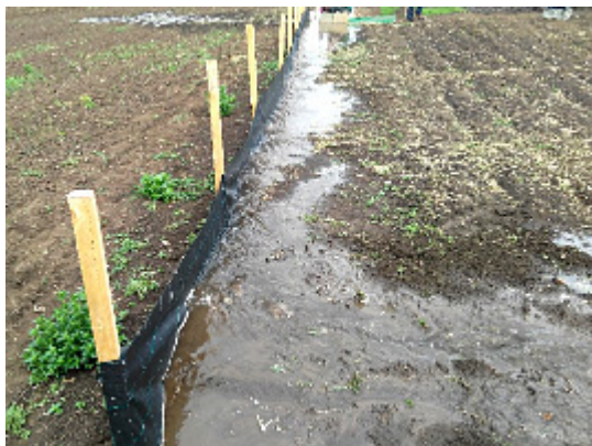
Figure S1. Directing run-off through the silt-fence barrier
