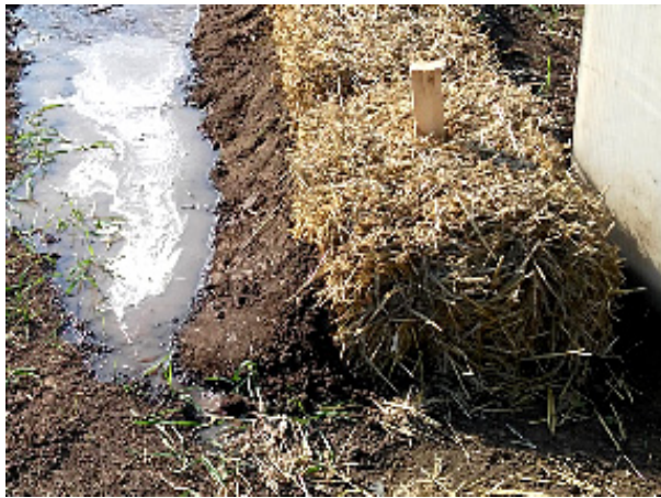
Figure S3. Profile of straw bale barrier
