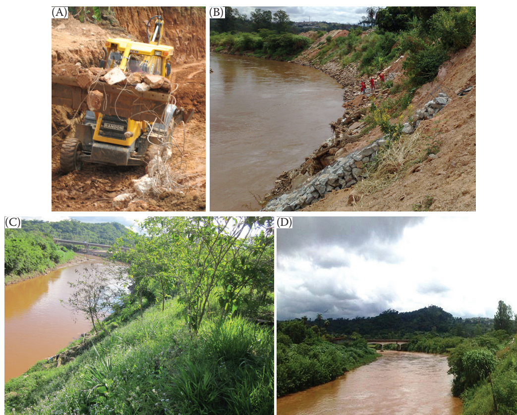
Figure 2. Slope rehabilitation: urban concrete construction wastes were used as fill at the base of the slope (A), slope before revegetation (B), slope 12 months after revegetation (C) and slope under flooding (D)
