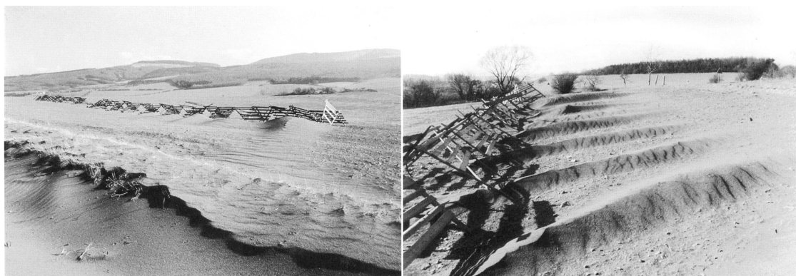
Figure 2. Spindle-shaped drifts transitioning into a road ditch covered by soil eroded by wind (Bánov 1990) – left; and spindle-shaped drifts with a pronounced ridge (Bánov 1990) – right (Švehlík 2002)
